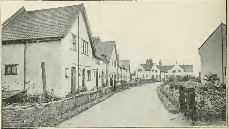
A VIEW OF EARSWICK, SHOWING ECONOMICAL ESTATE DEVELOPMENT.
