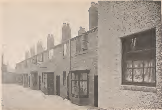
PHOTOGRAPH V.—ONE OF THE TERRACES AFTER THOROUGH REPAIR.
